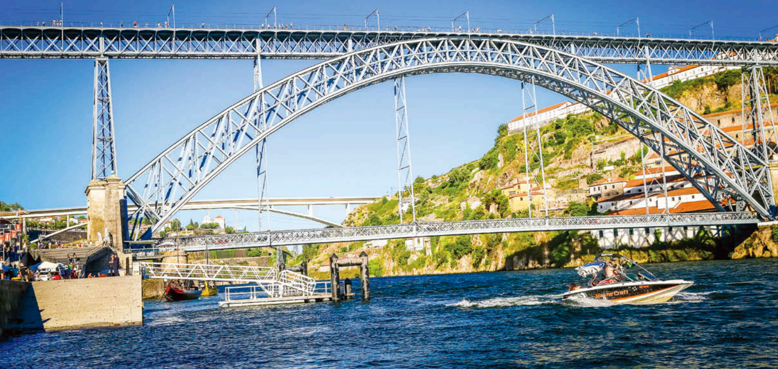
The Dom Luis metal arch bridge spans the Duoro River. Originally built in 1886, the upper level is a track for electric trains, while the lower level is shared by cars and pedestrians.
