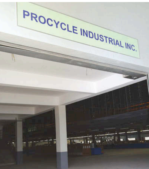
▲ Procycle's third plant is about 80% complete, and due to be fully completed by the end of September.
