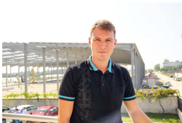
▲ Leader 96’s General Manager, Dimitar Zlatanov is standing in front of the under-construction new plant.
