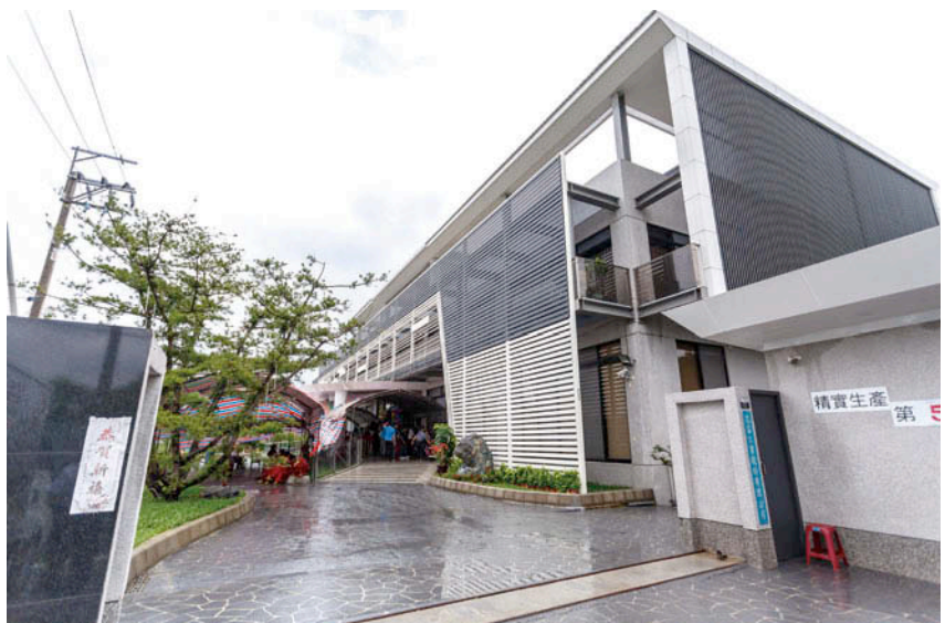
▲ King Roof's headquarters building has a green architectural design.
